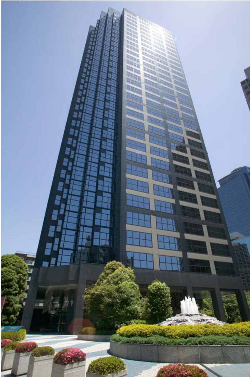
Photograph of the Shinjuku Square Tower
