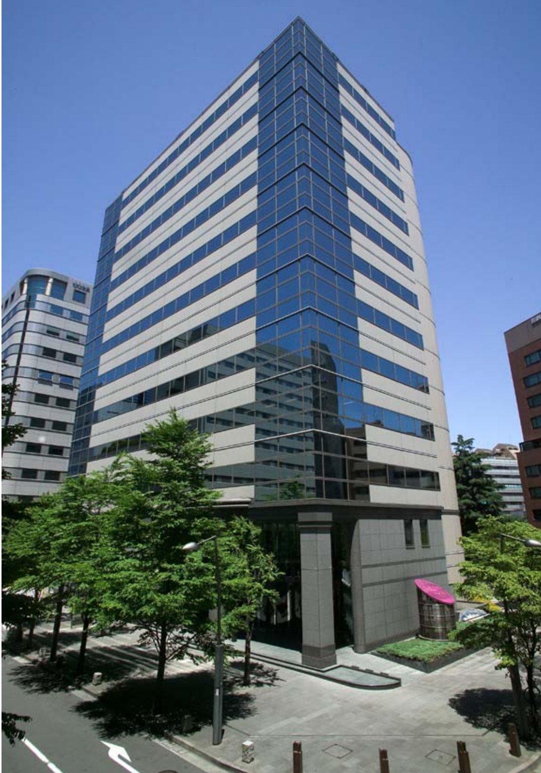
Photograph of the Tachikawa Business Center Building
