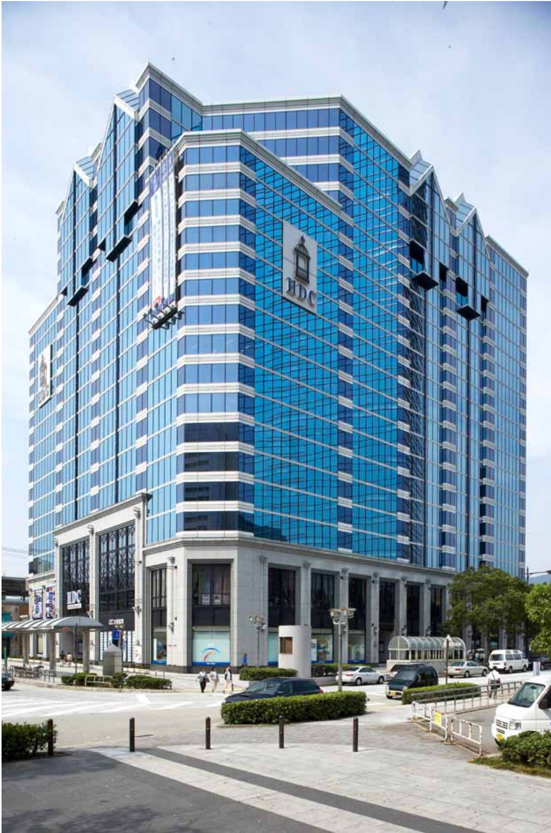
Photograph of the HDC Kobe
