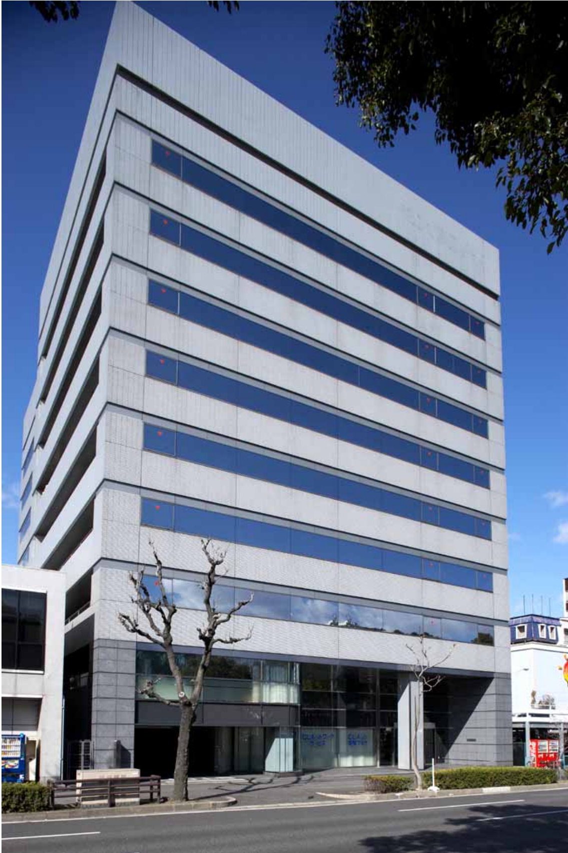
Photograph of the UFJ Central Leasing Head Office Building
