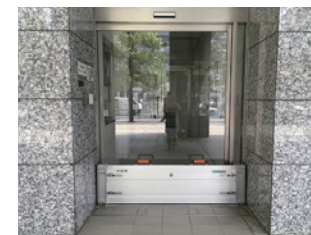
Olinas Tower 1F north exit passage
