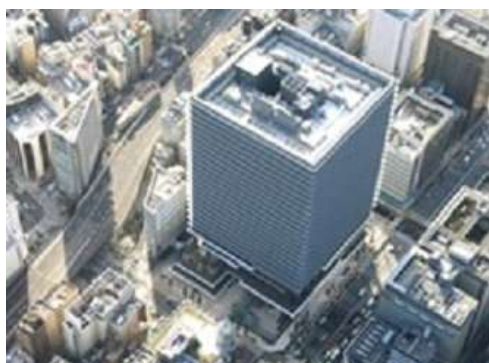
Tokyo Square Garden (Roof top)
