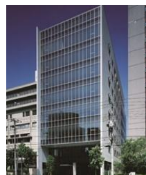
Shinagawa Canal Building
