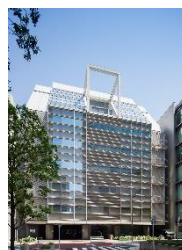
Kanematsu Bldg. Annex
