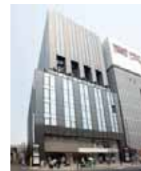
C-5 JPR Chayamachi Building
