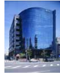
B-7 JPR Ueno East Bldg.
