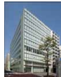
A-20 JPR Nihonbashi-horidome Building
