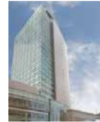
B-10 Yume-oka Office Tower
