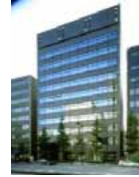
A-8 Fukuoka Bldg.
