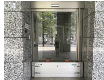
(Service entrance on the first floor of Olinas Tower)
