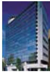
JPR Crest Takebashi Bldg.
