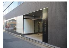
JPR Ningyocho Bldg. Renovation of the entrance
