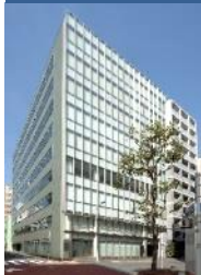
A-20 JPR Nihonbashi-horidome Building
