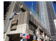
JPR Musashikosugi Bldg. Renovation of exterior walls
