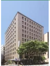
B-3 JPR Yokohama Nihon Odori Bldg.
