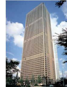
Shinjuku Center Building
