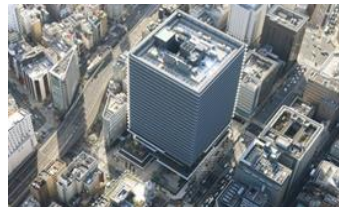
Tokyo Square Garden (roof)
