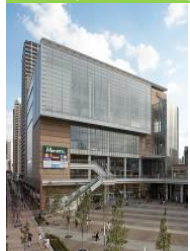
B-3 Cupo-la Main Bldg.
