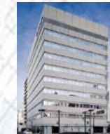
JPR Takamatsu Bldg.
