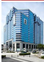
C-4 Housing Design Center Kobe
