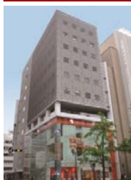
C-3 Benetton Shinsaibashi Bldg.
