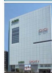
A-4 Shinjuku Sanchome East Bldg.
