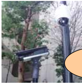
Installation of security cameras
