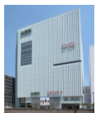
Shinjuku Sanchome East Building
