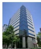
Tachikawa Business Center Building
