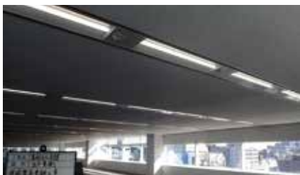
Replacement of lighting equipment with LED lamps in exclusive areas of Kanematsu Bldg.
