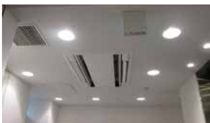
Replacement of air-conditioning units in elevator halls of JPR Shinsaibashi Bldg.
