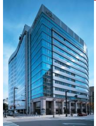
C-14 Tenjin 121 Bldg.
