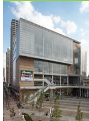
B-3 Cupo-la Main Bldg.
