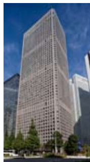
Shinjuku Center Building
