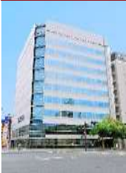
C-13 Sompco Japan Wakayama Bldg.
