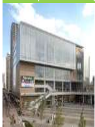
B-3 Cupo-la Main Bldg.
