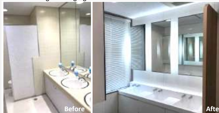
<JPR Naha Bldg. Building Age: 27 Years Toilets in common-use areas>
