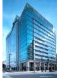
C-14 Tenjin 121 Bldg.
