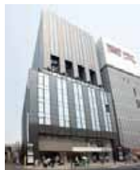
C-5 JPR Chayamachi Building
