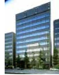
A-8 Fukuoka Bldg.
