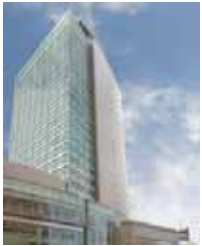
B-10 Yume-oka Office Tower
