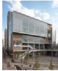
B-3 Cupo-la Main Bldg.
