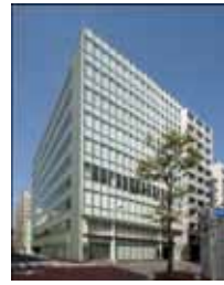
A-20 JPR Nihonbashi-horidome Building
