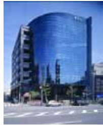
B-7 JPR Ueno East Bldg.
