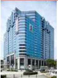
C-4 Housing Design Center Kobe
