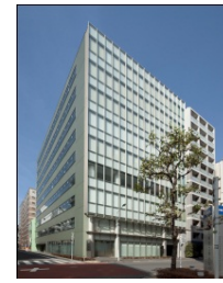
A-20 JPR Nihonbashi-horidome Building
