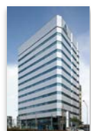
Shinyokohama 2nd Center Bldg.
