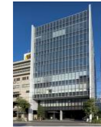
A-16 Shinagawa Canal Building
