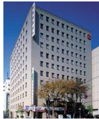
B-3 JPR Yokohama Nihon Odori Bldg.
