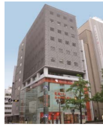
C-3 Benetton Shinsaibashi Bldg.
