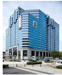
C-4 Housing Design Center Kobe
