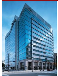
C-14 Tenjin 121 Bldg.
