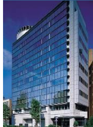
A-5 JPR Crest Takebashi Bldg.
