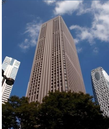
A-14 Shinjuku Center Building
