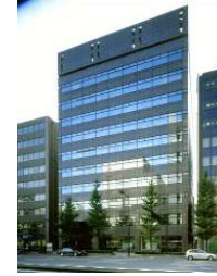
A-8 Fukuoka Bldg.
