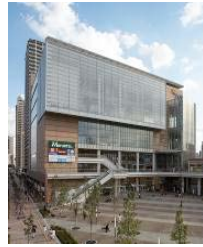
B-3 Cupo-la Main Bldg.
