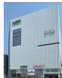
A-4 Shinjuku Sanchose East Bldg.
