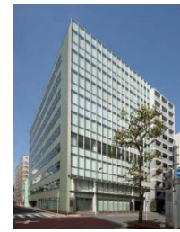
A-20 JPR Nihonbashi-horidome Building
