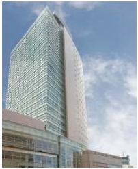
B-10 Yume-oka Office Tower
