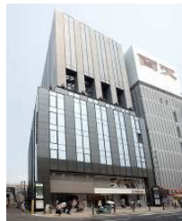
C-5 JPR Chayamachi Building
