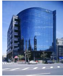
B-7 JPR Ueno East Bldg.
