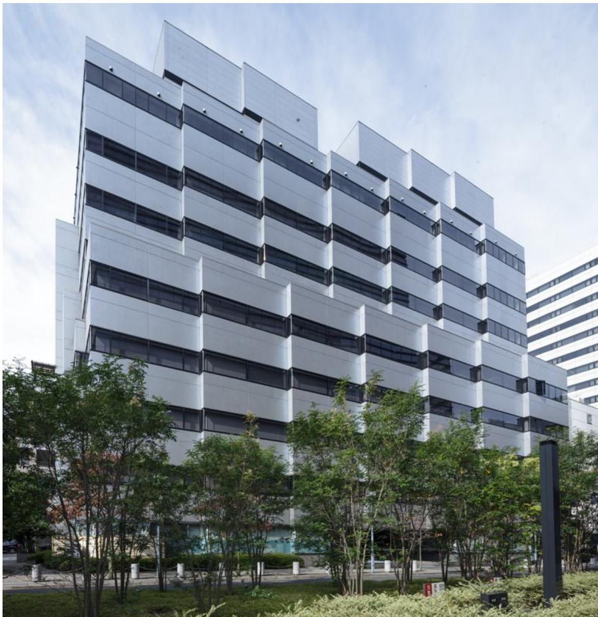
Photograph of Shibadaimon Center Building
