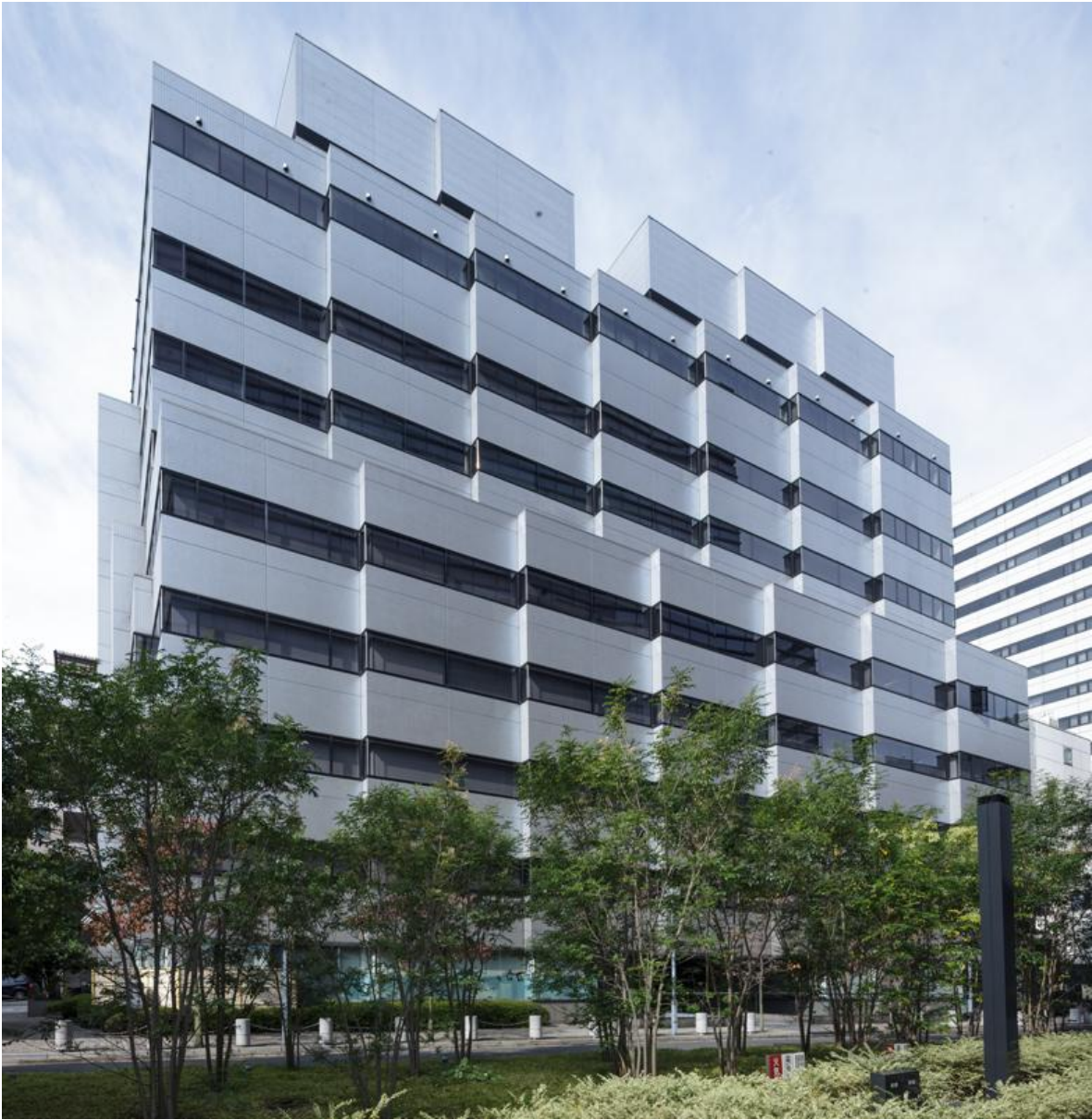
Photograph of Shibadaimon Center Building
