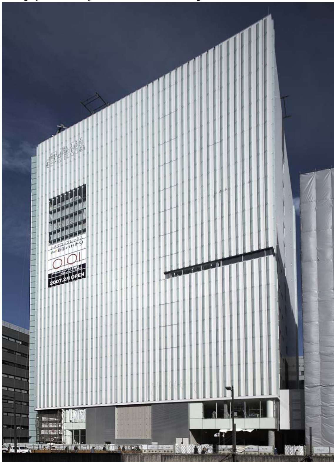
Photograph of the Shinjuku Sanchome East Building
