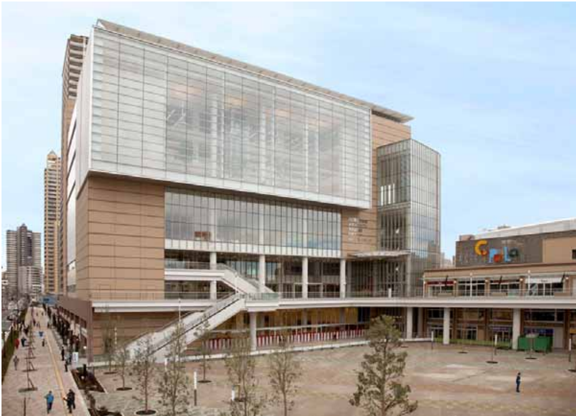
Photograph of the Cupo-la Main Building
