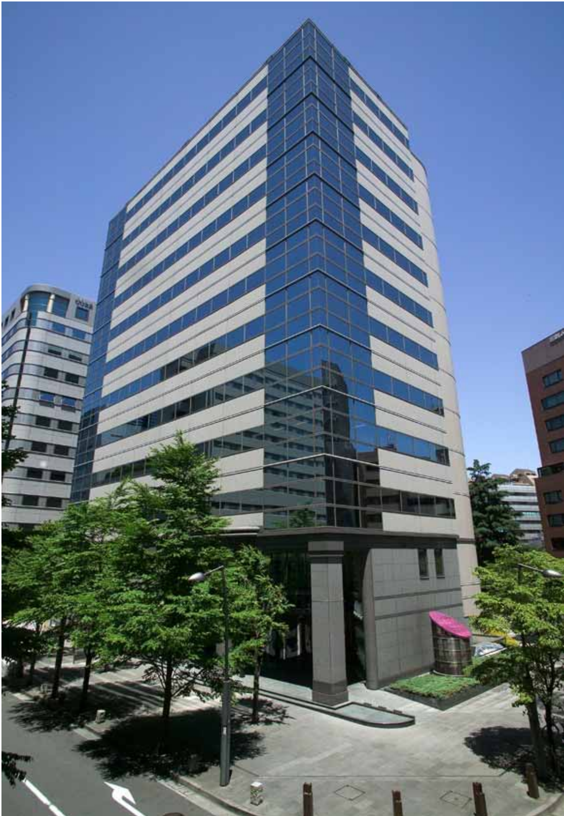
Photograph of the Tachikawa Business Center Building
