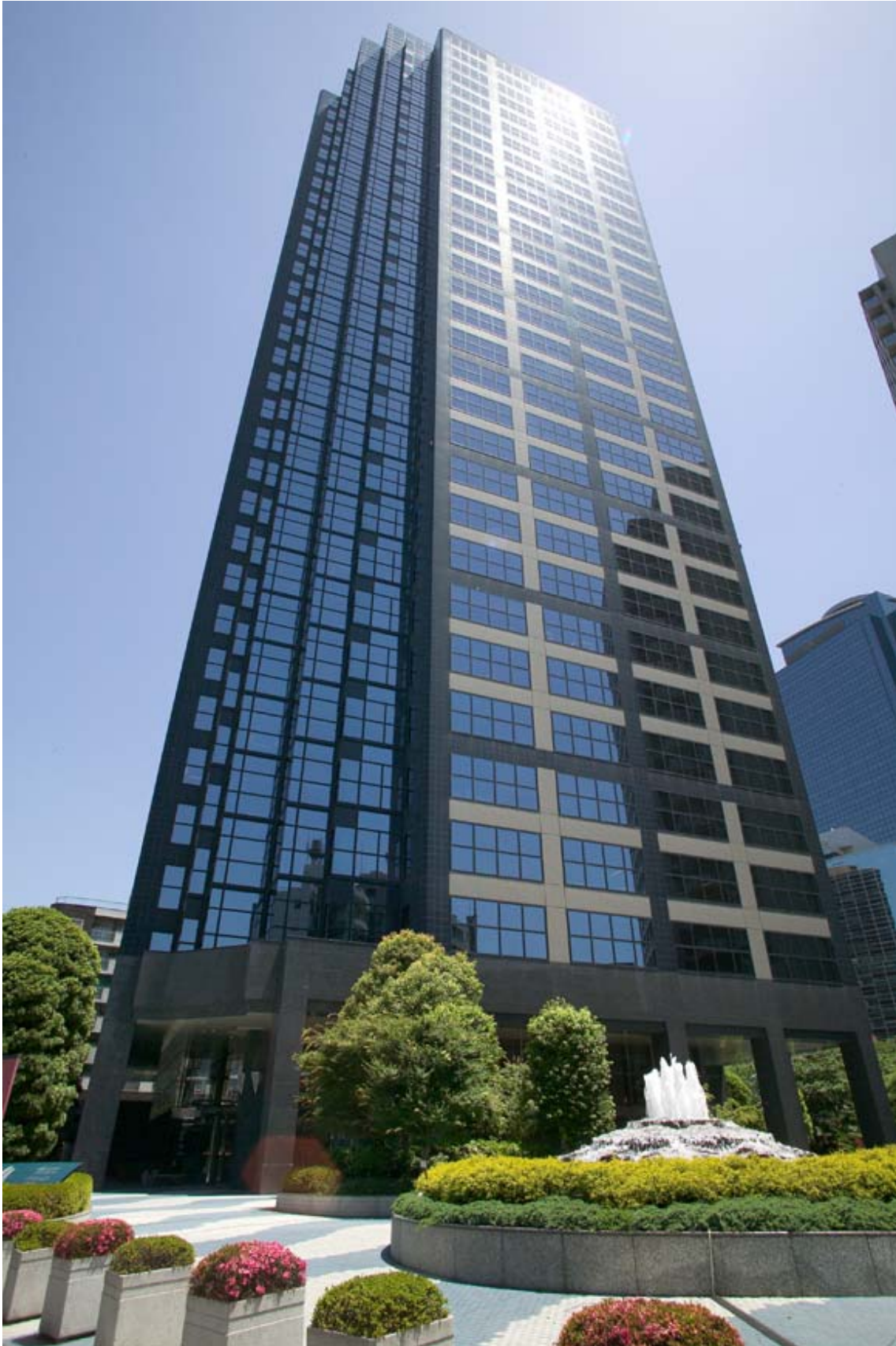
Photograph of the Shinjuku Square Tower
