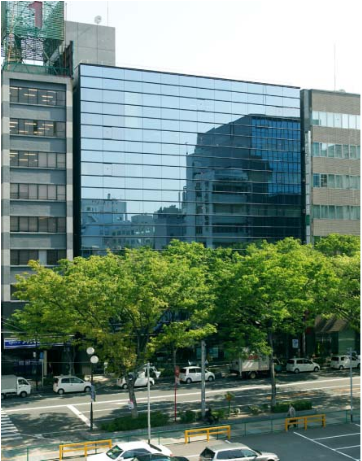
Photograph of the Semba Fukuoka Building
