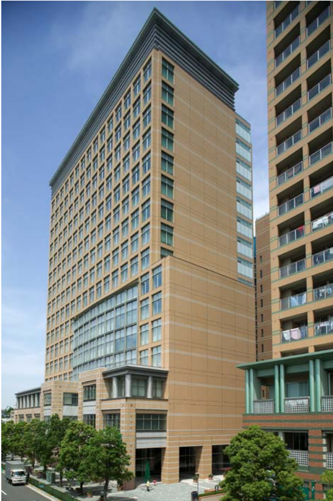
Photograph of the Oval Court Ohsaki Mark West
